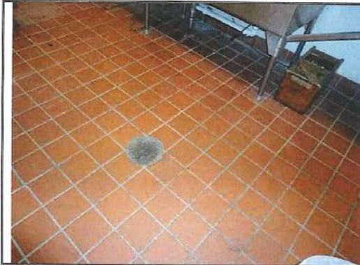
Photo 25 Basement (Kitchen floor drain)
