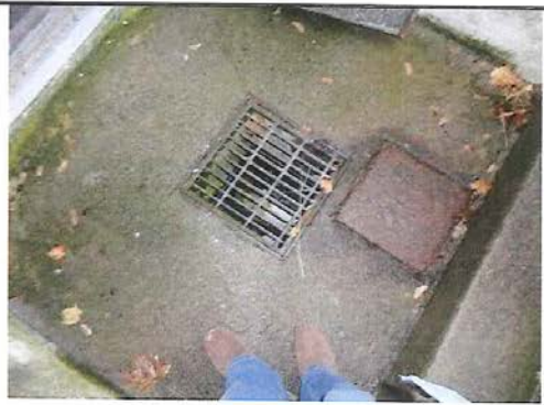
Photo 28 Storm Drain in exterior stairwell
