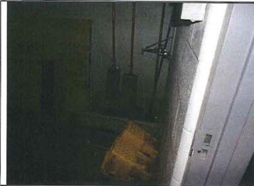
Photo 23 Basement (Custodial room)
